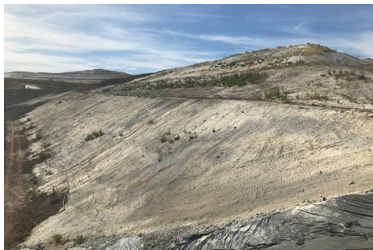
6 Months after application, site received over 11 inches of rain, and the Posi-Shell ® EC coating remains intact.
