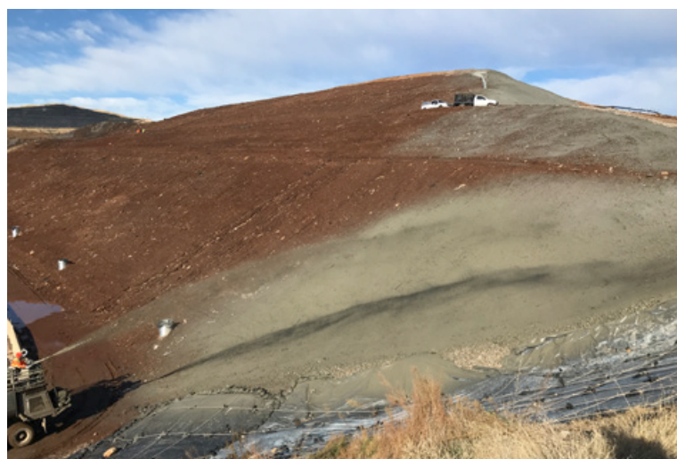
Posi-Shell ® EC application on the landfill's 2:1 slope.
