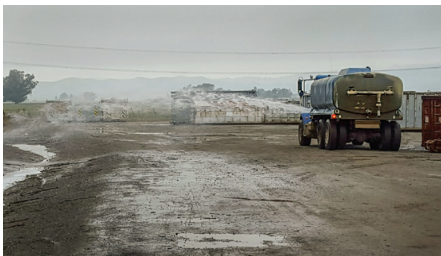
EarthGuard® was applied to the entire 1 acre site in under 1 hour with a standard water truck.
